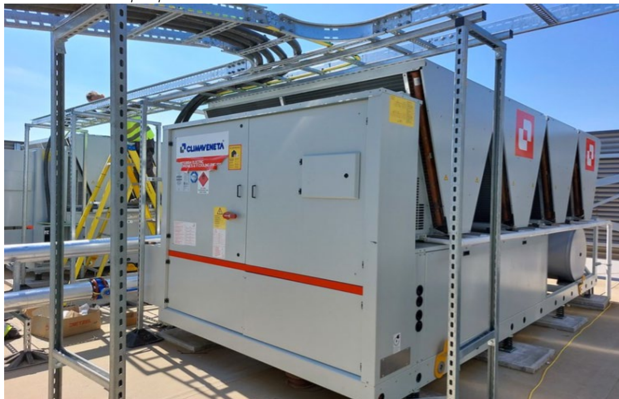
New air-source heat pump at Rivermead Leisure Centre
